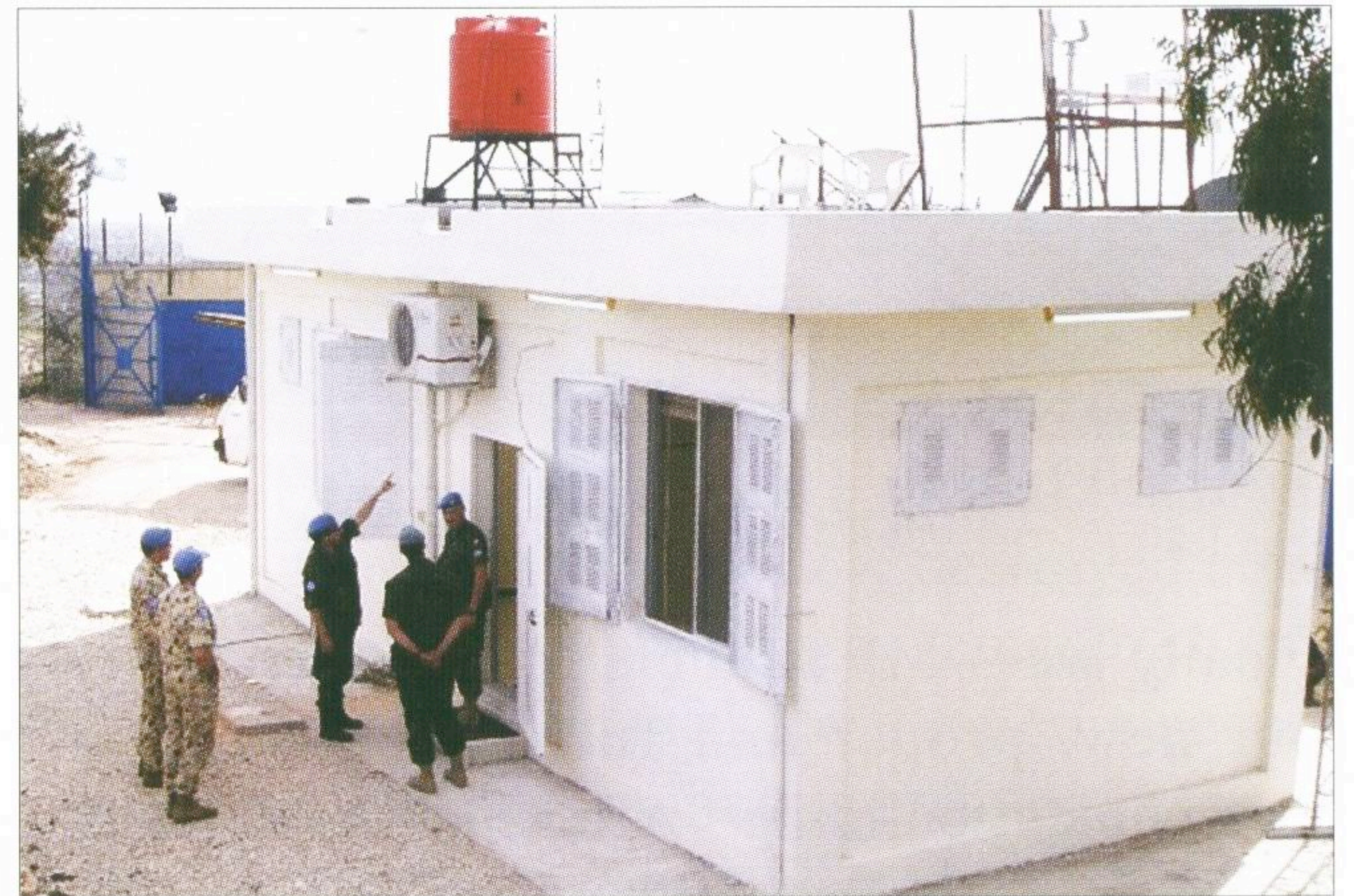
New accommodation OP 72
