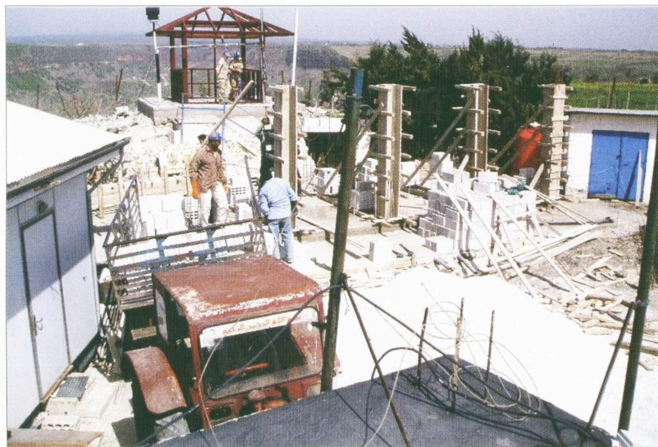
Work in full progress at OP 52
