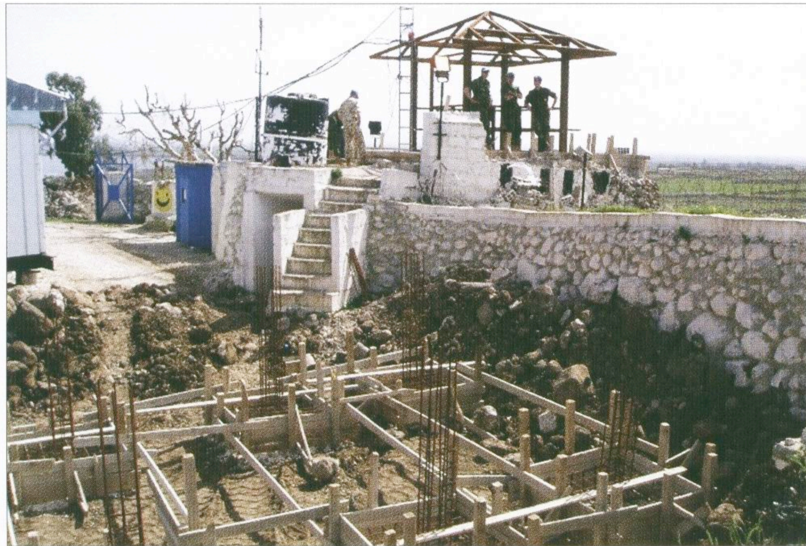
Preparations for the new accommodation and watchtower at OP 57
